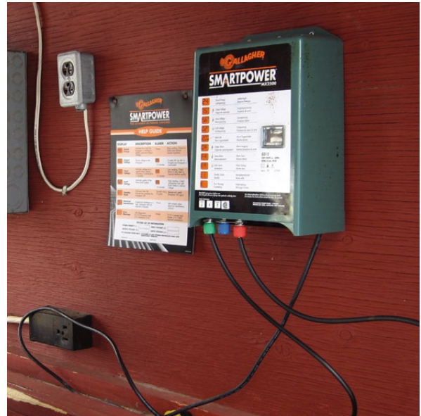
FIGURE 6 Electric fence charger installation
