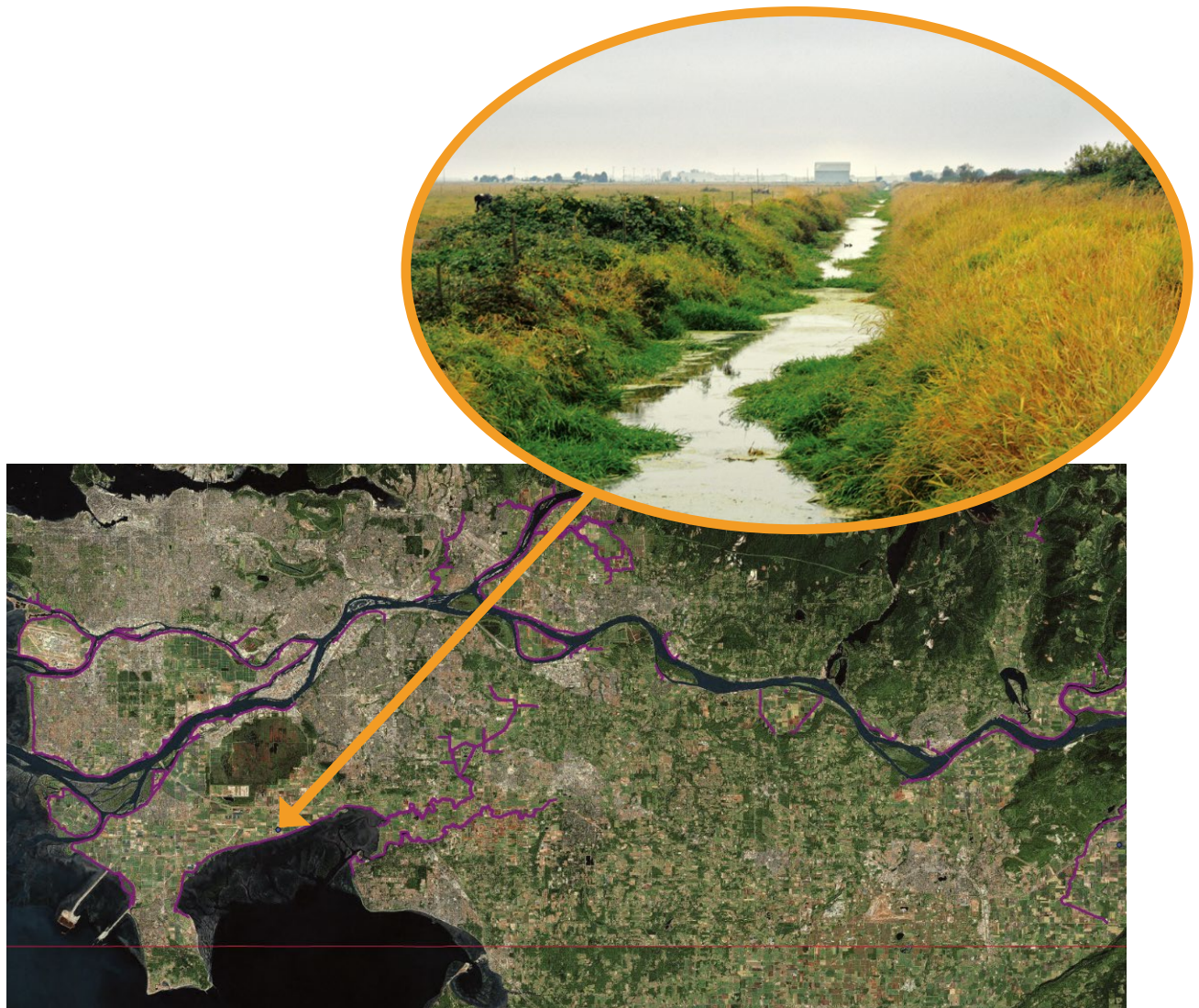
Constructed drainage ditch in the Fraser delta, in the very dry fall of 2012. The aerial map shows regional flood control works (linear features shown in purple).
