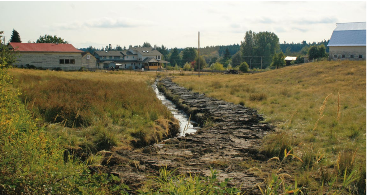
FIGURE 1 Surface drainage ditch in the Cowichan Valley
